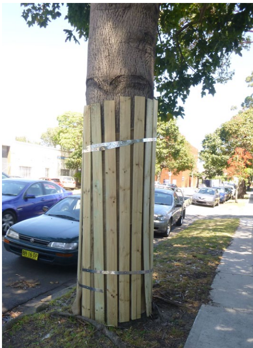
Figure 5.2 – Example of a temporary trunk protection (L) and ground protection (R) to be installed during construction periods. This can be a very valuable way of ensuring tree health and preventing accidental trunk damage and compaction of ground or disturbance of roots when work is undertaken close to trees. (Photo: Arterra)
