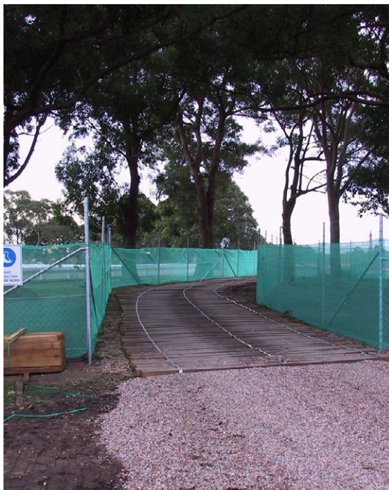
Figure 5.2 – Example of a temporary trunk protection (L) and ground protection (R) to be installed during construction periods. This can be a very valuable way of ensuring tree health and preventing accidental trunk damage and compaction of ground or disturbance of roots when work is undertaken close to trees. (Photo: Arterra)
