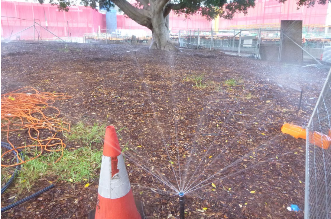
Figure 5.3 – Example of a temporary irrigation system provided to trees during construction periods. This can be a very valuable way of ensuring tree health and vitality is maintained and also promote new fibrous root growth closer to the trees. (Photo: Arterra)
